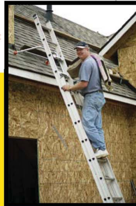
OSHA compliant roof access.
