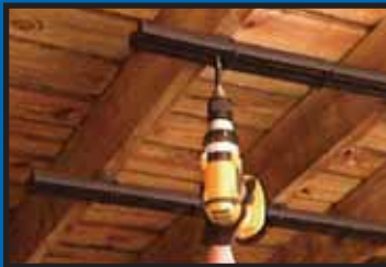
Screw joist brackets with pitch spacers attached into joist.
