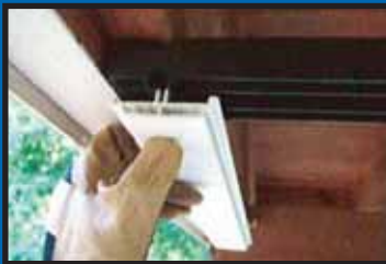
Snap starter channel to joist bracket.
