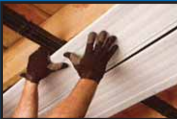
Snap panels into place and finish with trim cap
